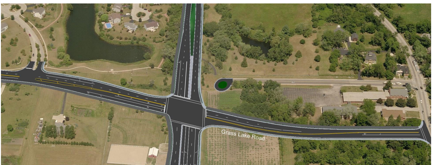
Looking North Along U.S. 45/Millburn Bypass at Grass Lake Road
