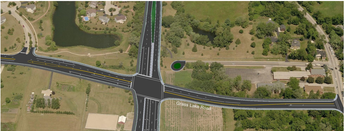
Looking North Along U.S. 45/Milburn Bypass at Grass Lake Road
