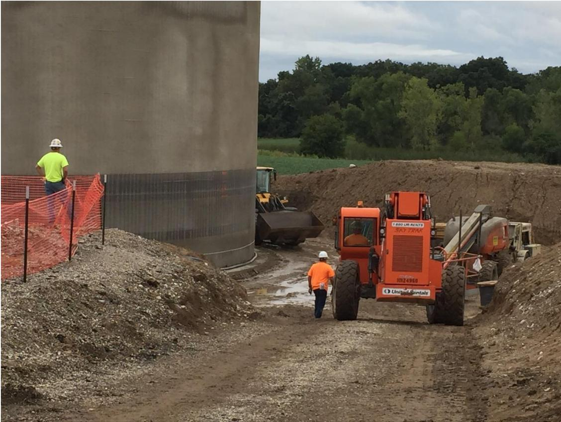
Steel Reinforcing Cable wrapped around the bottom of the reservoir
