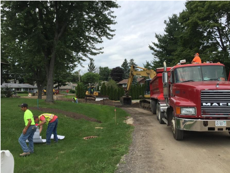
Road Base Preparation on Hickory Drive
