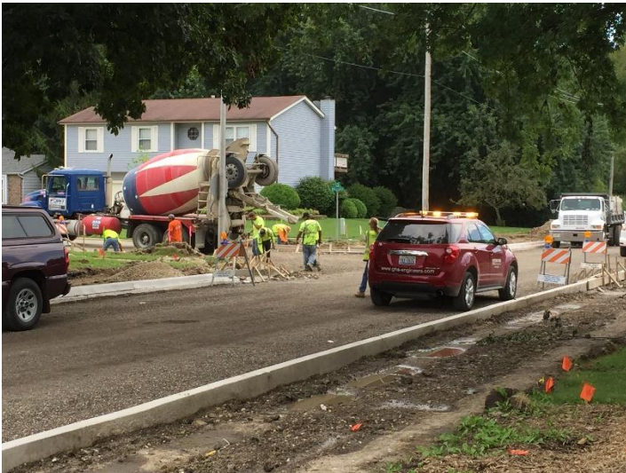
Concrete Work at Beck Road and Mallard Drive
