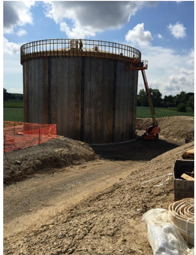
Before the Concrete was sprayed.
