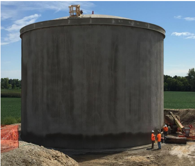
First Application of Spray Applied Concrete
