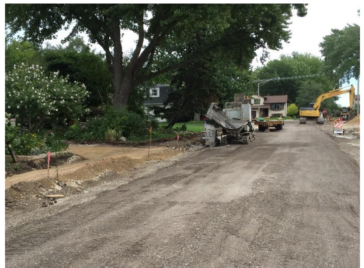
Curb and Gutter Slipforming on 2300 Block
