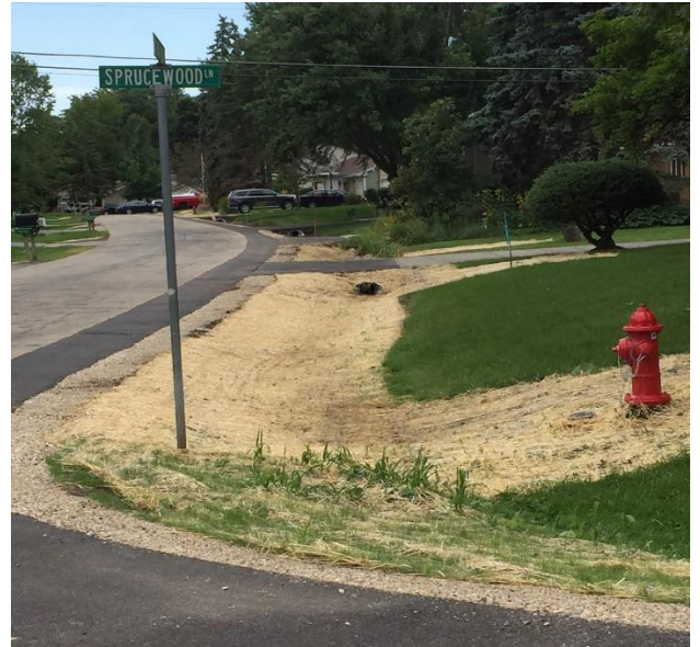
Rolling Ridge Lane Ditchwork
