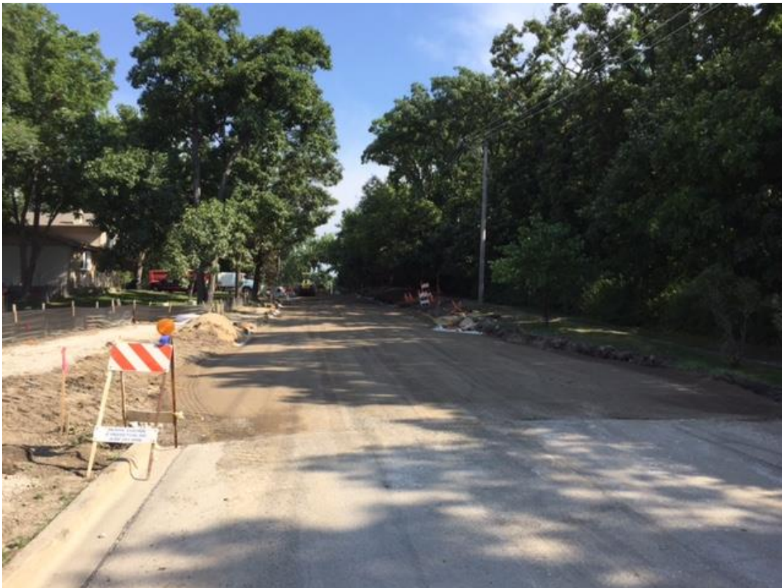
Beck Rd. looking north from Kelsey Road - base course placement
