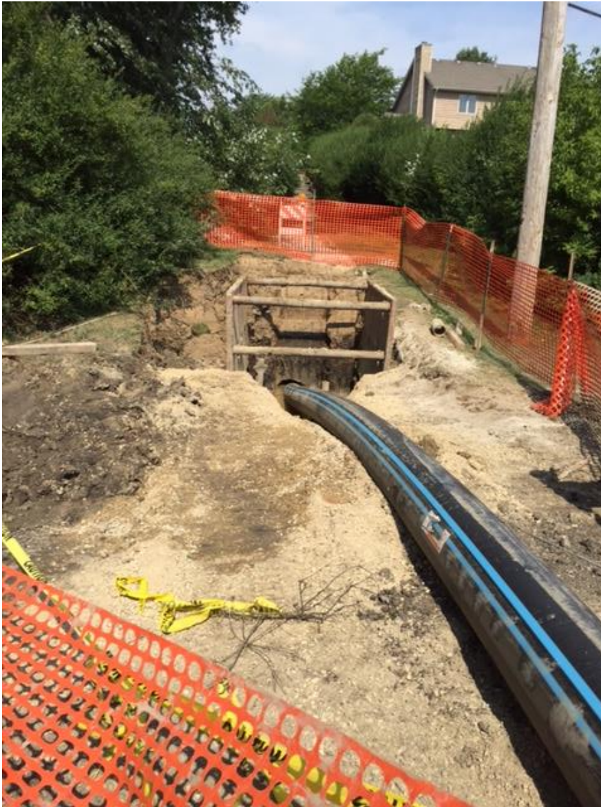
Hickory Ct, Directional drilling operation
