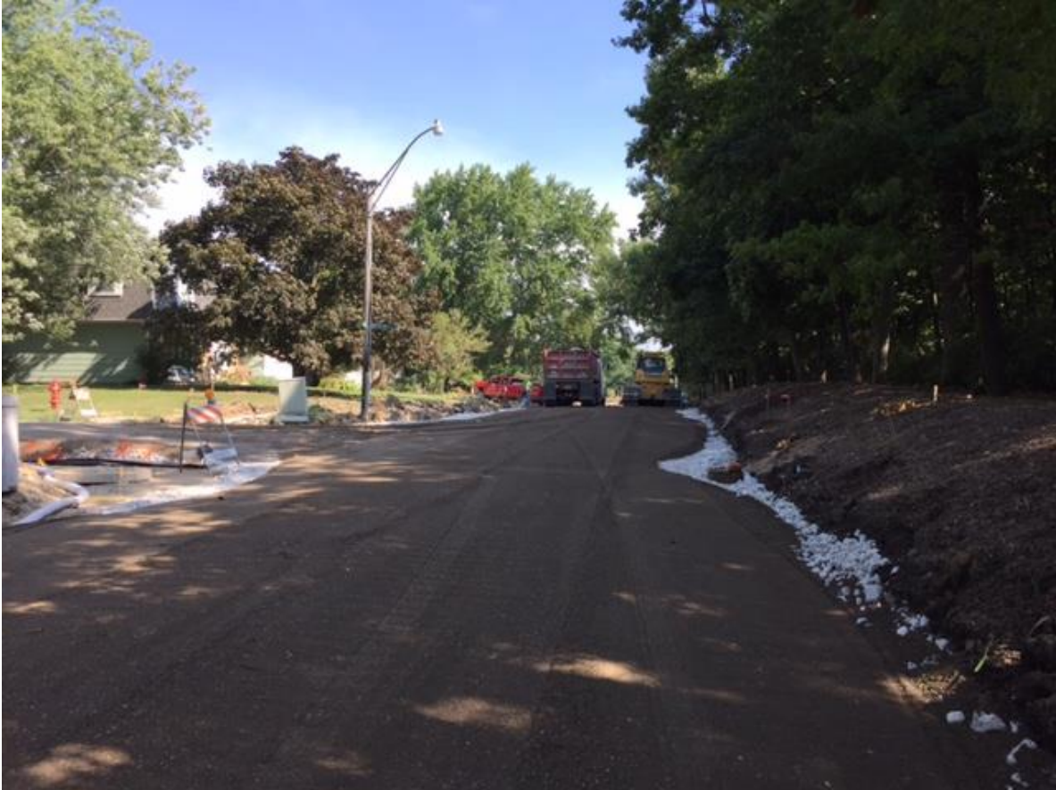
Beck Rd at Springhill- base placement
