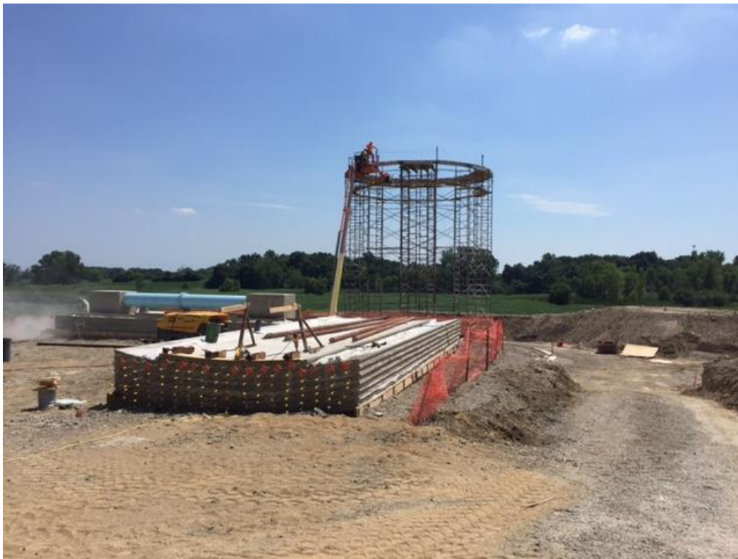
Pre-Cast sections (foreground) and scaffolding for reservoir in background.
